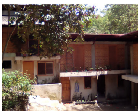
Housing Construction (PESTALES)
