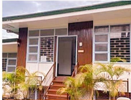
Renovations on new location (Balay Sofia)
